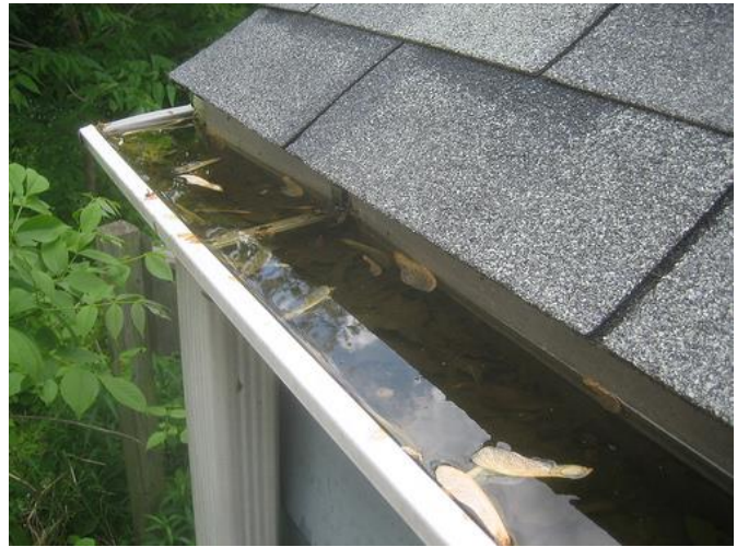
Figure 8. Clogged rain gutter filled with water
