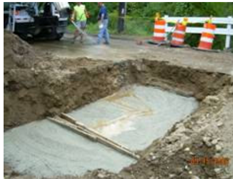
Repairs to culvert
