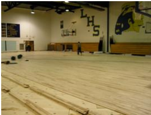
New resilient athletic hardwood floor being installed
