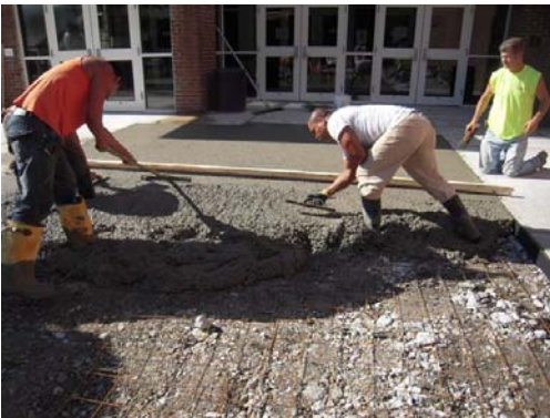
New Concrete sidewalk and ramp at High School
