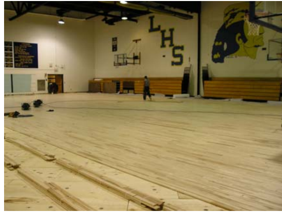
New resilient athletic hardwood floor being installed
