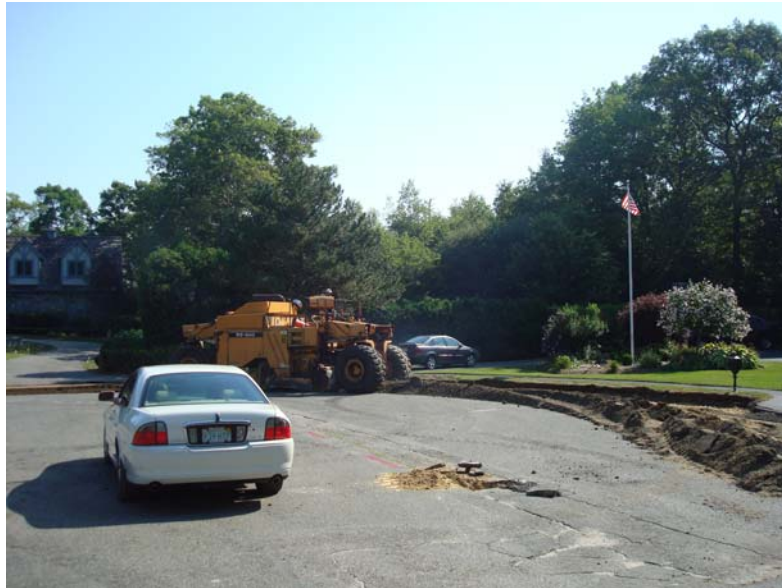
Reclamation of existing pavement- Magnolia Drive
