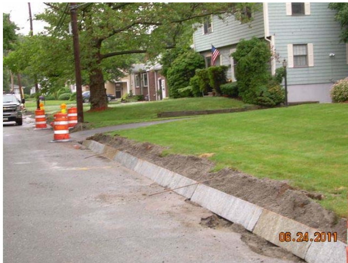
Setting sloped granite curb- Brook Drive
