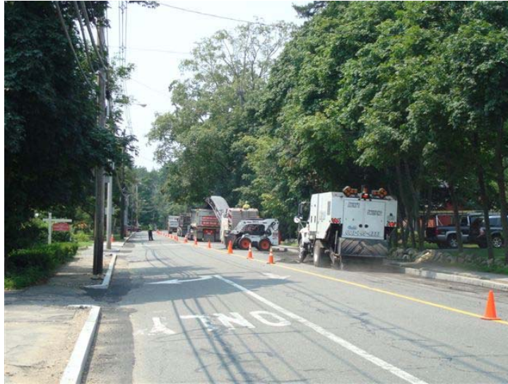
Milling existing pavement- Salem Street
