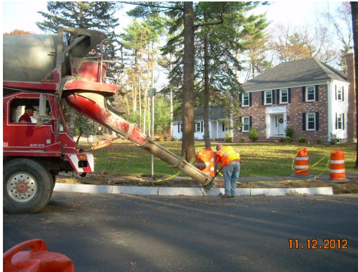
Installation of granite curbing on Durham Drive
