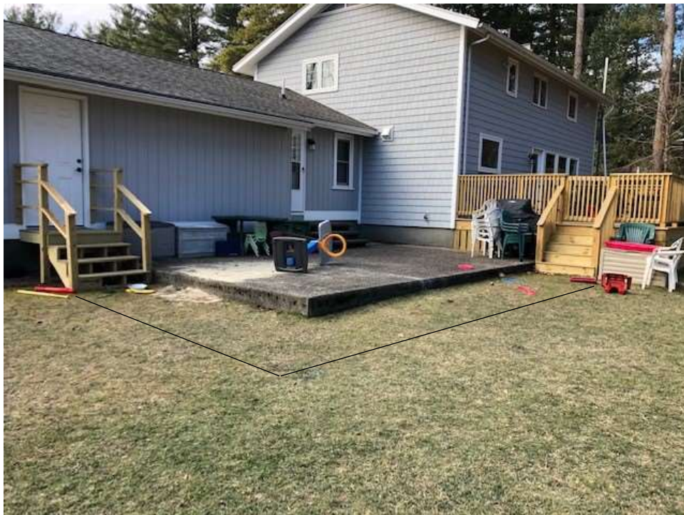
Photo 5 : Existing patio off rear of dwelling to be reconstructed and expanded by 4' to existing steps from deck and garage (as approximated by black lines).
