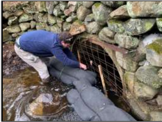
Figure 1 BioChar sock installation
