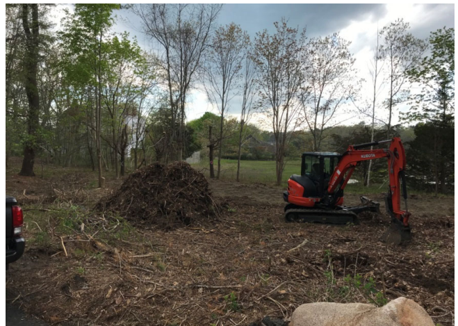
Whole Plant Removal techniques employed using a mini excavator
