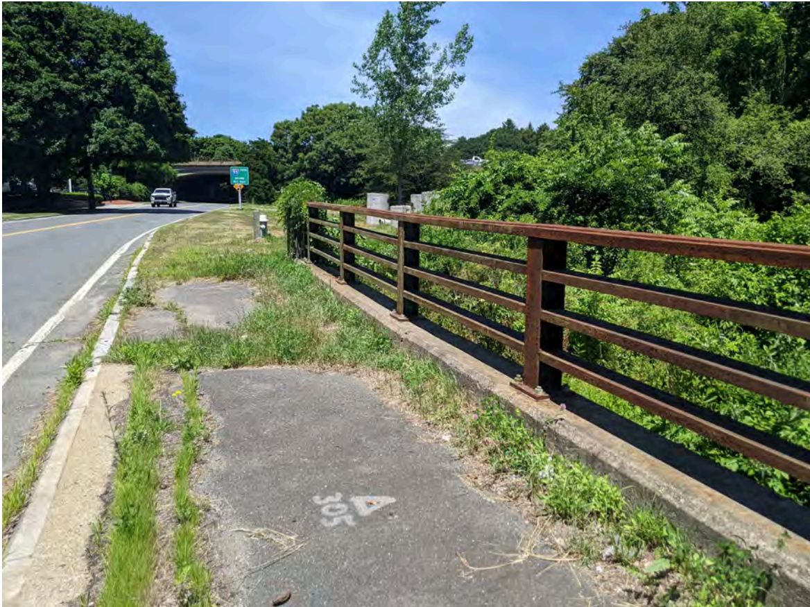
Figure 3. Saugus Bridge (Eastern Side)
