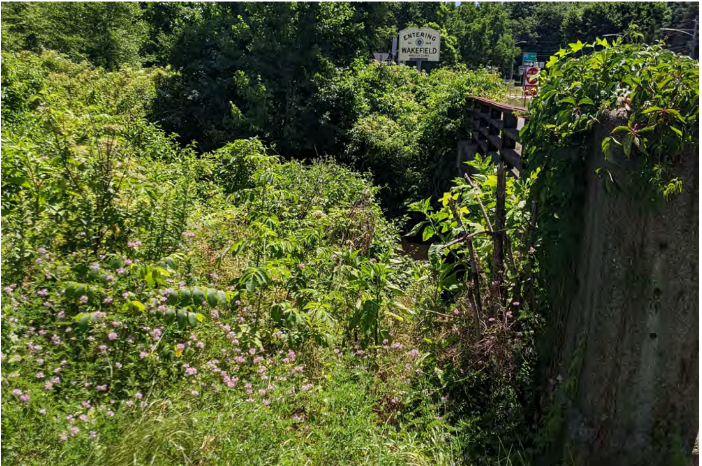
Figure 4. Saugus Bridge (Eastern Side)
