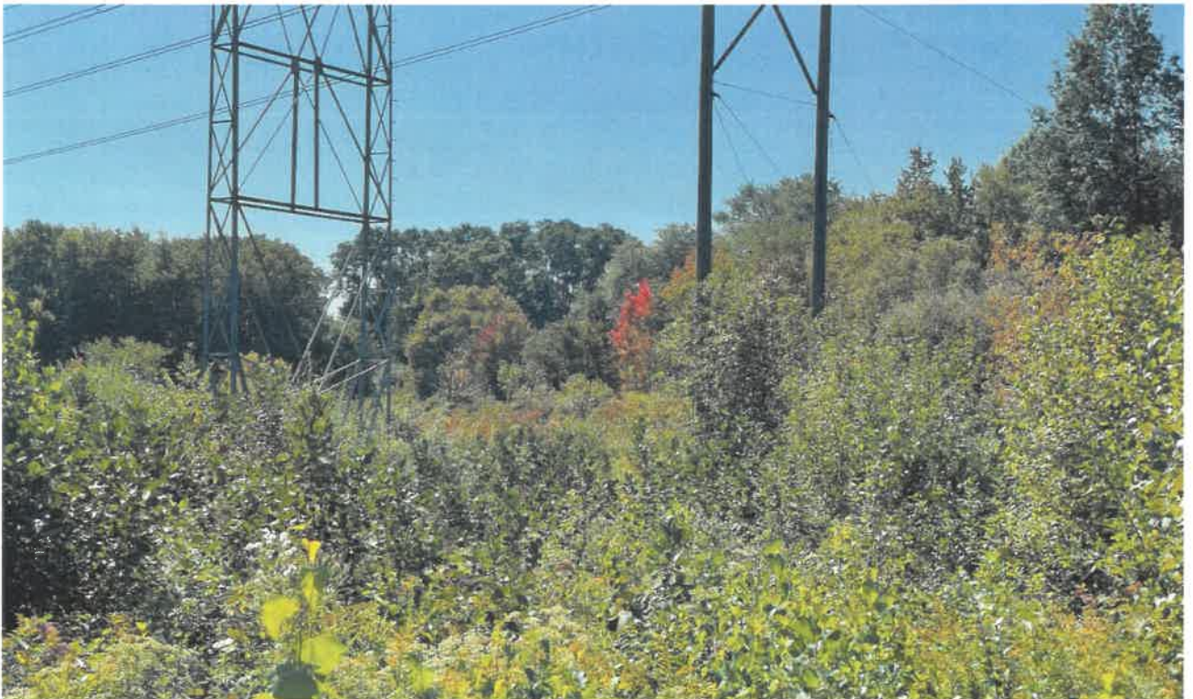
Photo #2: View of restored areas proximate to Structure 114. Facing north.
