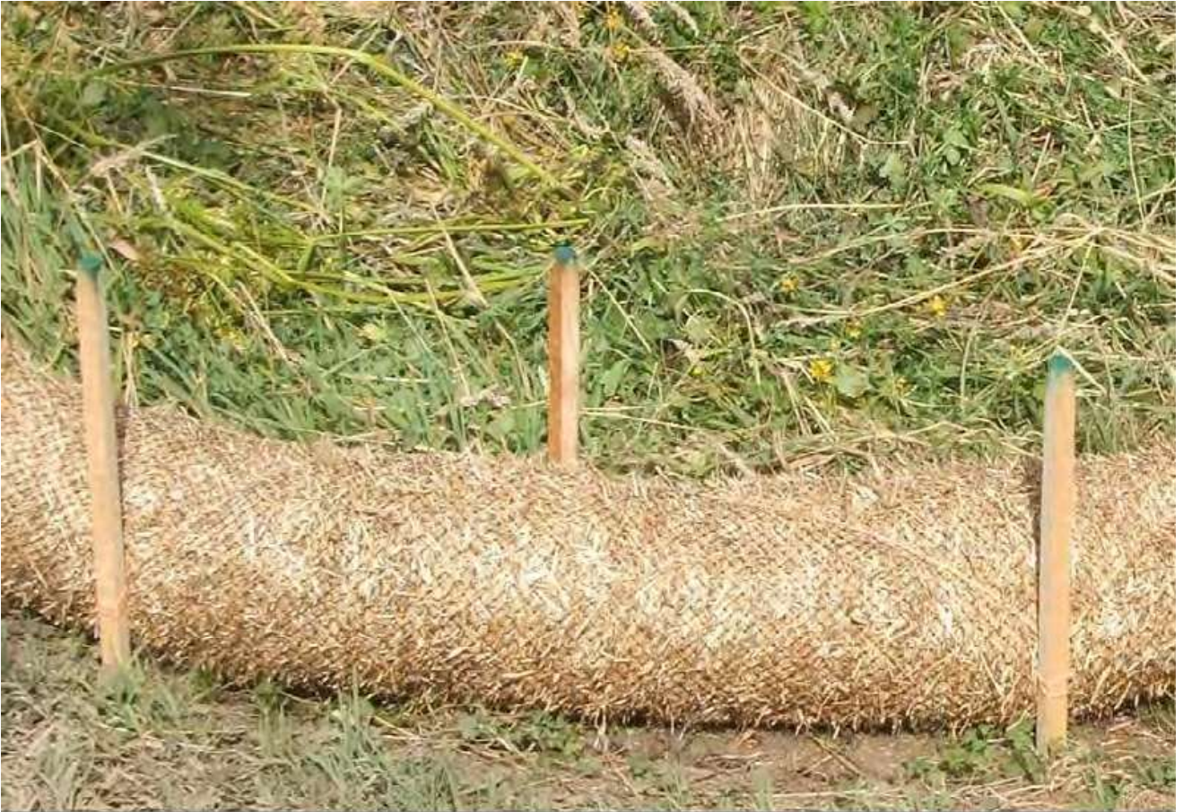
STRAW WATTLE – SHALLOW SLOPE ( \leq 4:1 ) (ALTERNATE STAKING)
