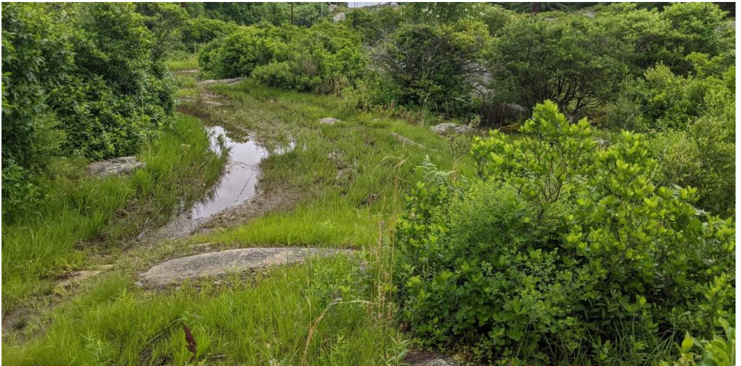
Photo #6: View of access to Structure 92 on the T146E Line and Structure 91 on the S145E Line, where the proposed access is within the BVW and 100-foot Buffer Zone looking east.
