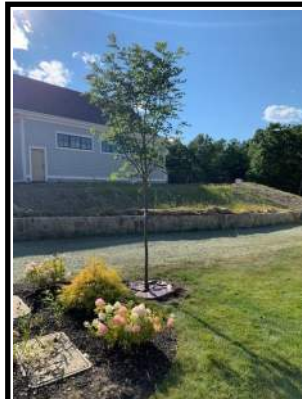
DRAINAGE EASEMENT STABILIZED & SEDIMENT FOREBAY
