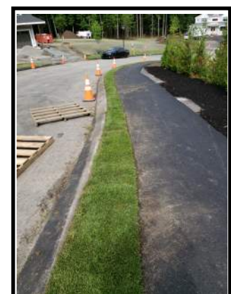
SOD PLANTED WITHIN SUBDIVISION R.O.W.
