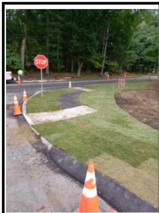
SOD PLANTED WITHIN SUBDIVISION R.O.W.
