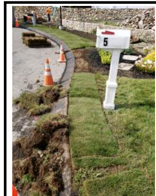
SOD PLANTED WITHIN SUBDIVISION R.O.W.
