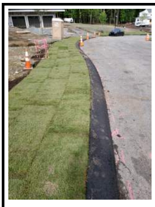
SOD PLANTED WITHIN SUBDIVISION R.O.W.
