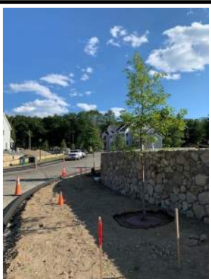
DRAINAGE EASEMENT STABILIZED & SEDIMENT FOREBAY
