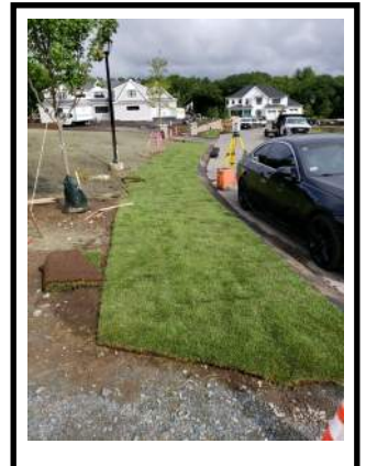
SOD PLANTED WITHIN SUBDIVISION R.O.W.
