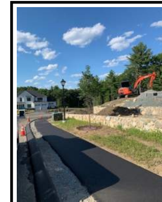
NEW ASPHALT BERM & FINISH PAVEMENT ON SIDEWALK
