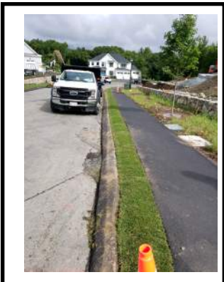
SOD PLANTED WITHIN SUBDIVISION R.O.W.
