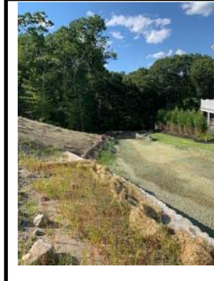
DRAINAGE EASEMENT STABILIZED & SEDIMENT FOREBAY
