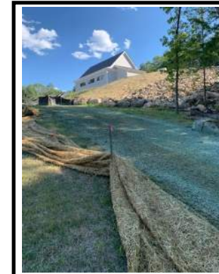
DRAINAGE EASEMENT STABILIZED & SEDIMENT FOREBAY
