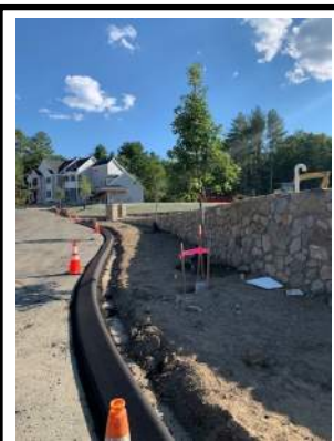
NEW ASPHALT BERM & FINISH PAVEMENT ON SIDEWALK
