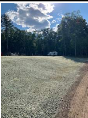
# 2 SAGAMORE BONDED FIBER MATRIX STABILIZATION & SWALE
