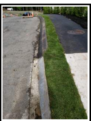
SOD PLANTED WITHIN SUBDIVISION R.O.W.
