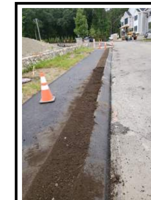
NEW ASPHALT BERM & FINISH PAVEMENT ON SIDEWALK
