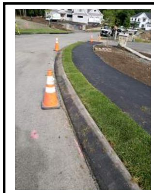
SOD PLANTED WITHIN SUBDIVISION R.O.W.
