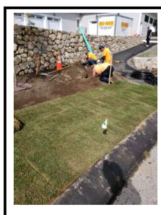
SOD PLANTED WITHIN SUBDIVISION R.O.W.
