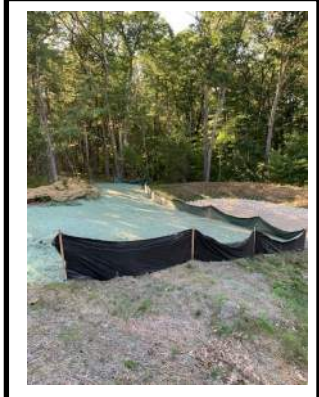
DRAINAGE EASEMENT STABILIZED & SEDIMENT FOREBAY
