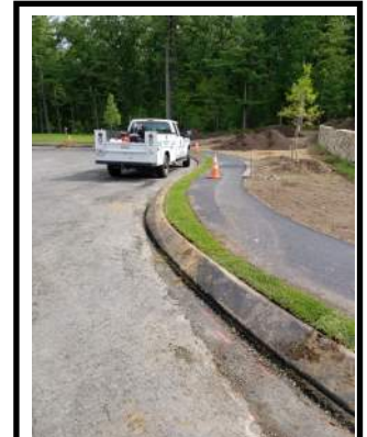
SOD PLANTED WITHIN SUBDIVISION R.O.W.
