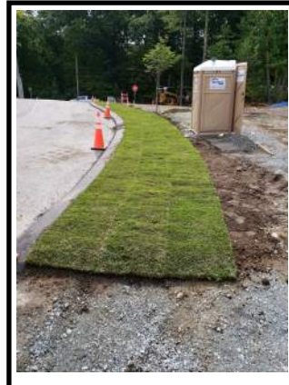
SOD PLANTED WITHIN SUBDIVISION R.O.W.
