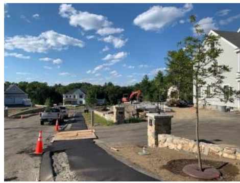
NEW ASPHALT BERM & FINISH PAVEMENT ON SIDEWALK
