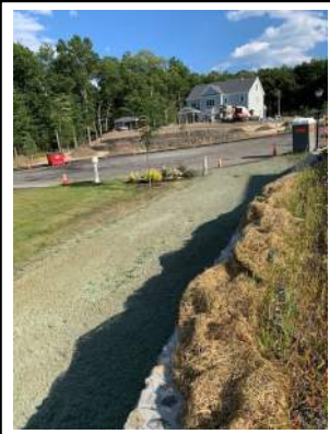
DRAINAGE EASEMENT STABILIZED & SEDIMENT FOREBAY
