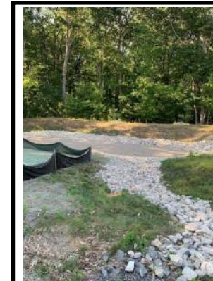
DRAINAGE EASEMENT STABILIZED & SEDIMENT FOREBAY
