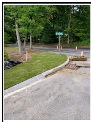
SOD PLANTED WITHIN SUBDIVISION R.O.W.
