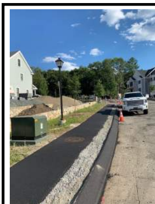
NEW ASPHALT BERM & FINISH PAVEMENT ON SIDEWALK
