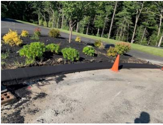
NEW ASPHALT BERM & FINISH PAVEMENT ON SIDEWALK
