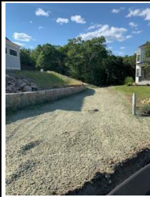
DRAINAGE EASEMENT STABILIZED & SEDIMENT FOREBAY
