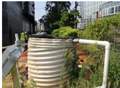
Figure 4. Dewatering discharge operations.
