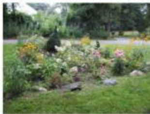
Rain garden — a shallow depression in the ground that collects stormwater, and can be planted with shrubs or flowers
