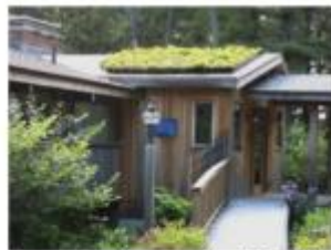
Green roof — one planted with vegetation that absorbs some of the rain that falls on it
