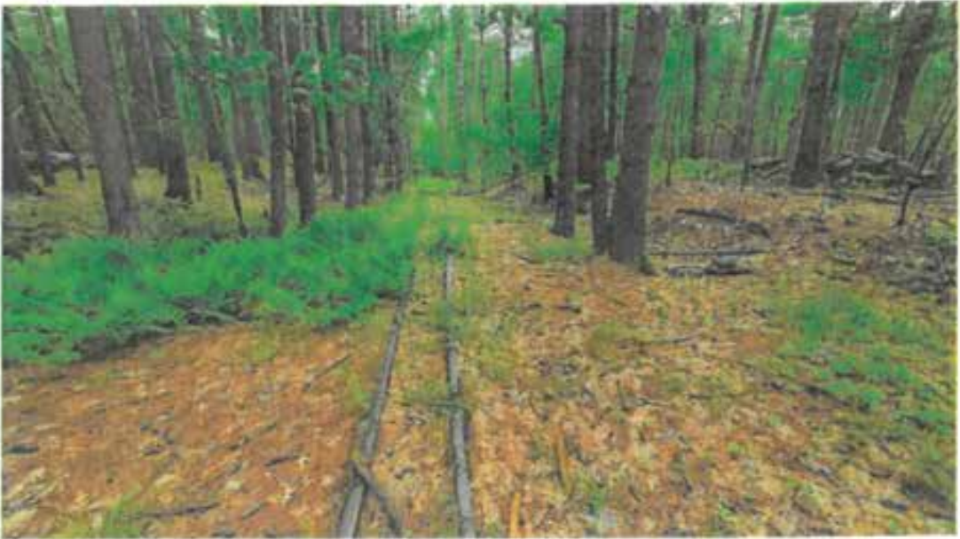
Photo 2. Old rails will need to be removed from a few hundred yards of the rail bed just west of the Bostik property.
